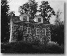
left was once a door. The lowpitched roof, stoned-up gable ends, and H/L hinges on the interior doors are other indications of a later, more Americanized style of house.
